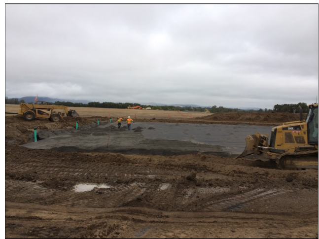
EcoRain Inspection/Cleanout Portal Tanks were installed.
