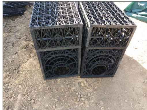
EcoRain Inspection/Cleanout Portal Tanks were installed.
